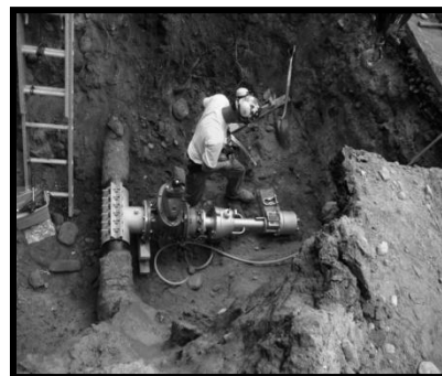
Contractor installing a "Tapping Sleeve" and Gate Valve to connect the new water main on Wheeler
